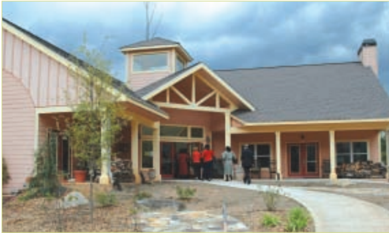
People with physical disabilities can easily enter the “visitable” clubhouse at East Lake Commons, a town home community in Decatur. Renovating a home to be visitable can cost thousands, but building one from scratch might cost just a few extra dollars for a wider doorframe and door.
