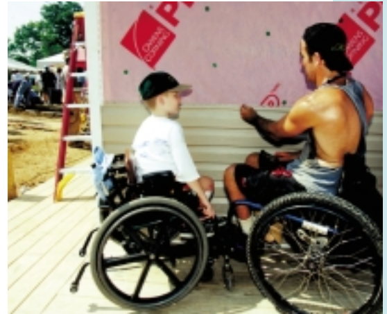
Volunteers with disabilities worked alongside volunteers from BellSouth and BellSouth Telecom Pioneers to complete the ABILITY House in only seven days of construction.
